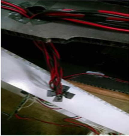
Figure 1: Current Solar Car Wire Usage
