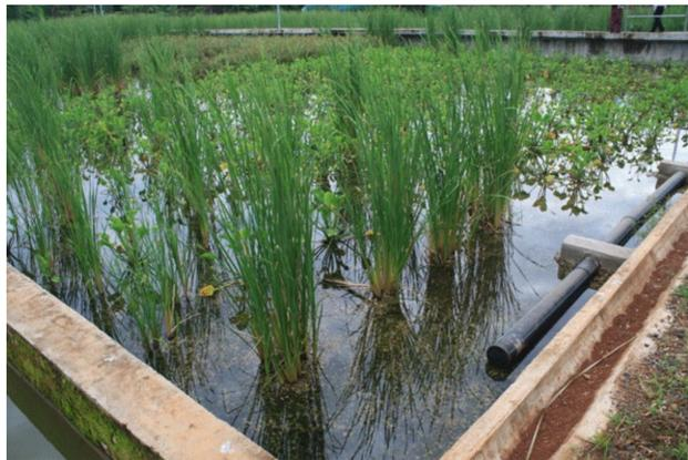
Figure 1: Photo of constructed wetland for use in wastewater treatment. Source: Adapted from [1]
