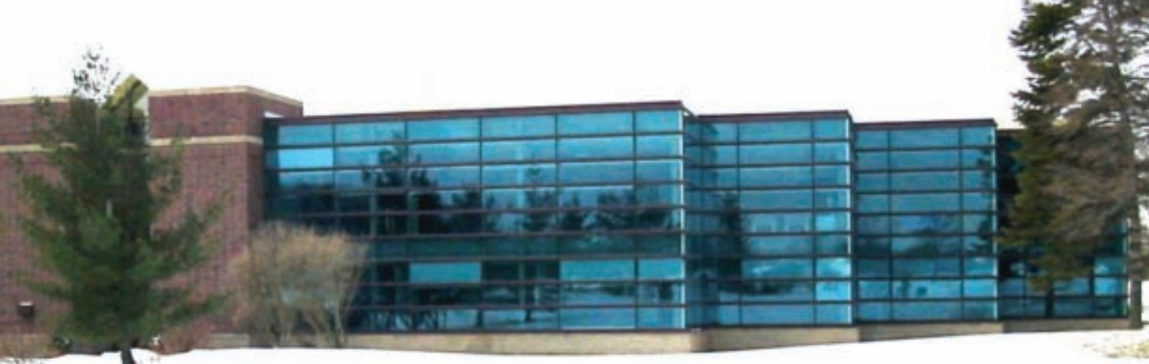
The home of the Composite Vehicle Research Center (CVRC).
