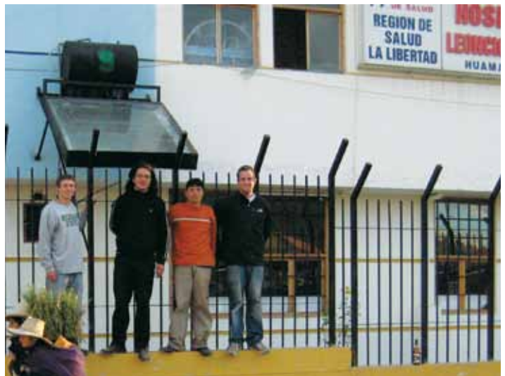
Mathieu Rich (right), an ME senior, and Austin Melcher (far left), a CHEMS junior, were helped by two Peruvians in establishing a solar water heater at a hospital in the northern Andean town of Huamachuco.
