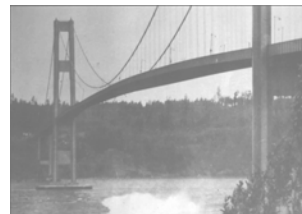
Wind-induced vibrations
